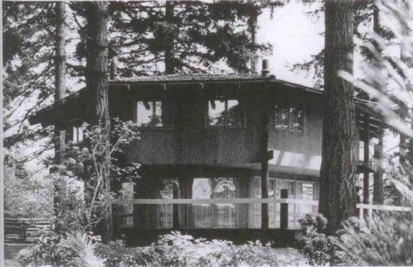
Figure 14-2 This octagonally shaped home is perfectly suited for location on a piece of high ground—perhaps a bluff or rolling hill—where breath-taking vistas surround the dwelling. The house shown has heavy beams supported by peeled poles and a massive stone fireplace to add drama to the living room. To keep exterior maintenance to a minimum, handsplit shakes
