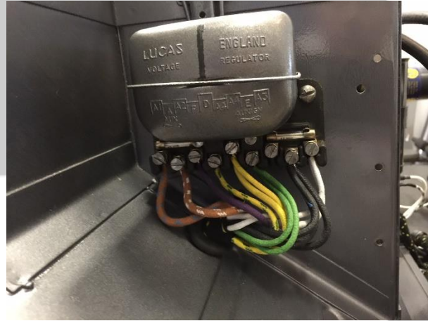
Brand New Wiring to Regulator
