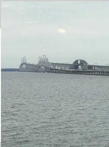
A cloudy day view of the magnificent Chesapeake Bay Bridge
